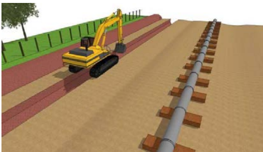
Figure 2.3 Trench Excavation
